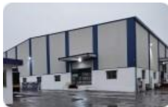
Chakan ART Facility
