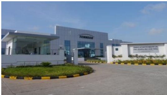
Chakan I Facility
